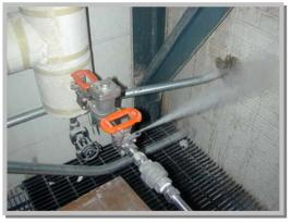
operation should be taken for evaluation, benchmarking and training purposes of proper steam trap operation.
